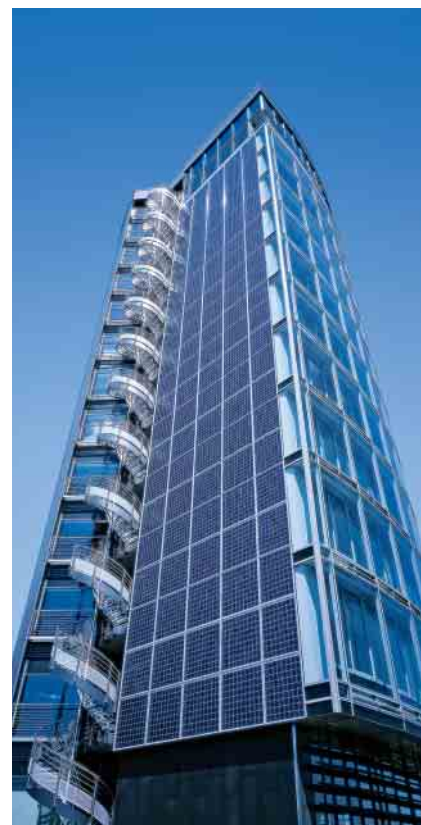
Bauerfeind Tower, Zeulenroda, Germany
