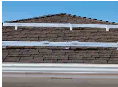
SolarEZ rails minimize roof penetrations.
